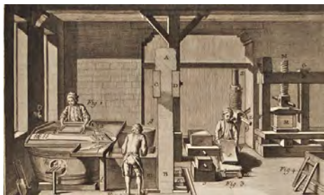
Handling by Vatman, Coucher, and Layer
