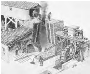
18C Charcoal Iron Blast Furnace
